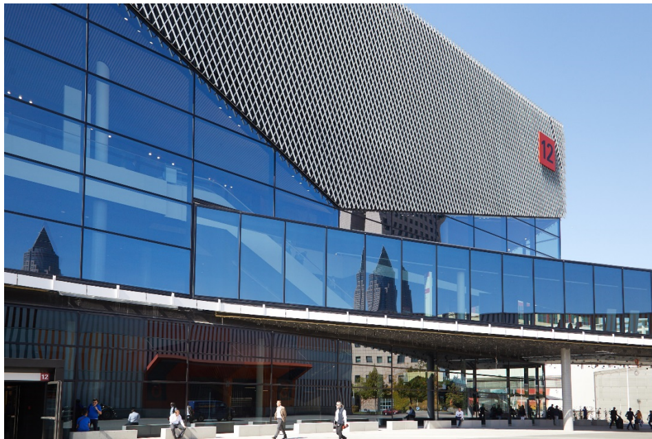
The new Hall 12 Source: Messe Frankfurt
